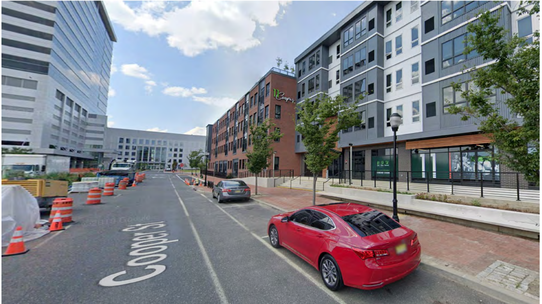
11 Cooper, built in 2019, is one of the most recent mixed-use residential developments in the area. The project added 156 market-rate and affordable units, as well as retail space on the ground floor level.
