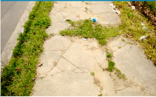
Poorly maintained sidewalks
