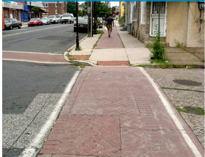
Commercial areas could be enhanced with basic public realm improvements, as seen in neighboring Pennsauken
