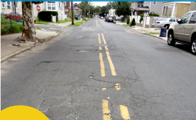
Poor roadway conditions on 27th Street
